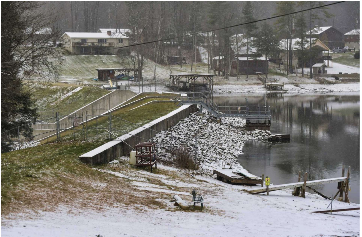
A view of the Hadlock Pond Dam on Dec. 8 in Fort Ann. A dam at this site failed in 2005; the dam was rebuilt in 2007. Paul Buckowski / Times Union
