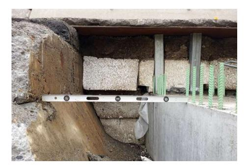
the white material is Styrofoam. yes you are driving on it, it fills the entire cavity of what was dugout between the old abutment and the hole opened up to set the new abutments- about 8" of fill on top of that and then 1" road plates as the driving surface, when a loaded tractor and trailer drove over this you could see the plate deflect about 3/4"
