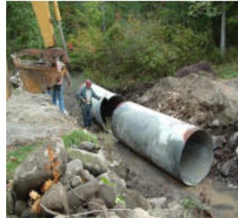
In October, the Crown Point Highway Department installed a new culvert at the base of the Ben Hunter Road! The new culvert is substantially wider and offers a more secure roadbed for those who live on, deliver and/or travel to the north side of Eagle Lake.
