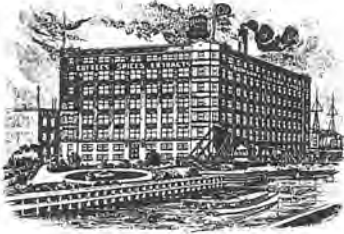
2219 ST. BRIDGE TELEPHONE CANAL 4000
