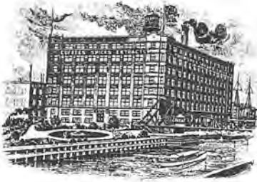
22 ND ST BRIDGE TELEPHONE CANAL 4000
